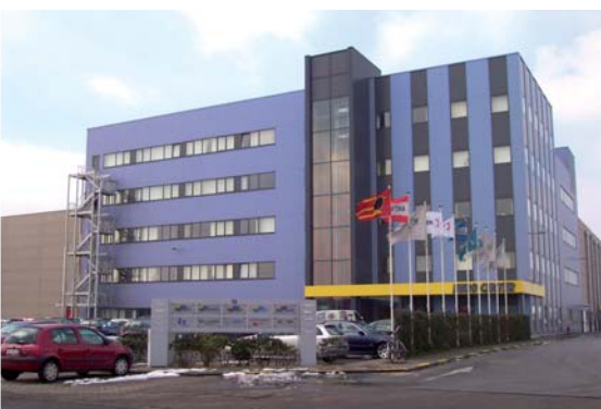
De Grave-Antverpia offices in Liège in Belgium
