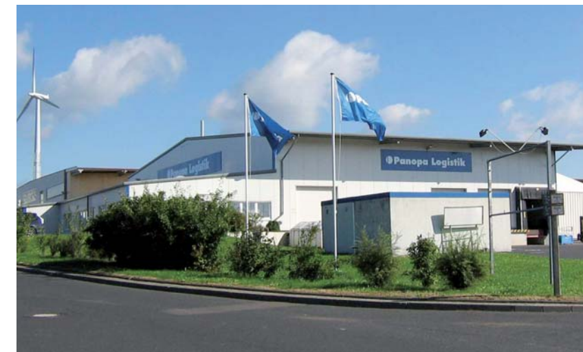
Front axle support preassembly and sequencing by 20 employees in Großenlupnitz
